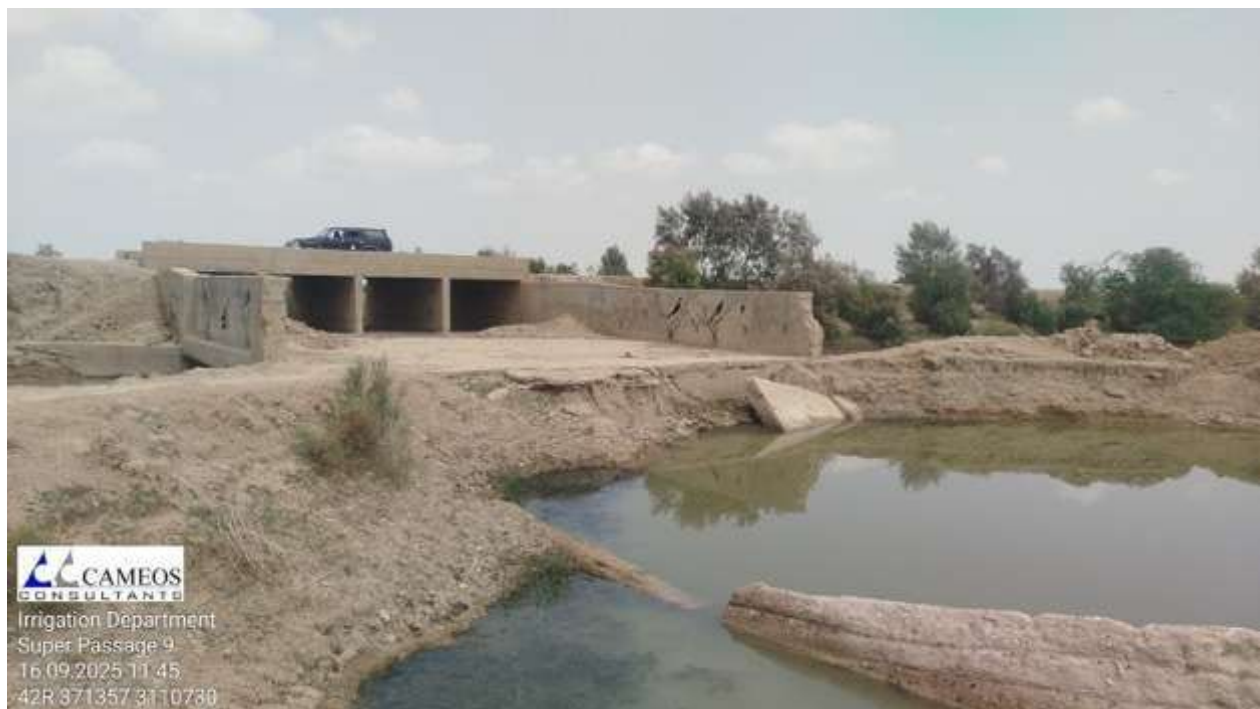
Figure-3-2: Alluvial/riverbed deposits along the washed-out Channel.
