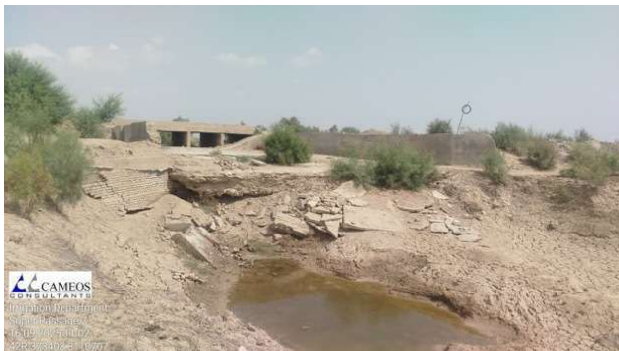
Figure-3-3: Alluvial deposits (Clayey Silt, Silty Clay and Gravelly Silt) along the sub-project site
