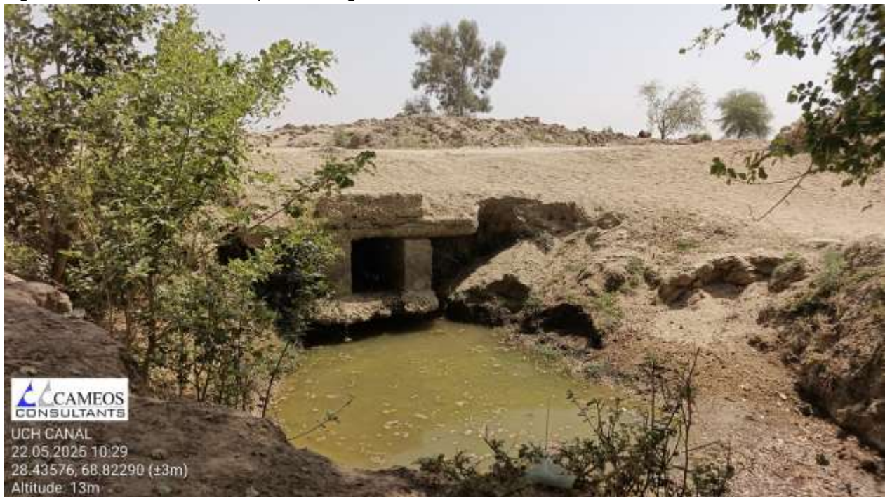
Figure-3-3: Alluvial deposits (Clayey Silt, Silty Clay and Gravely Silt) along the Uch canal.
