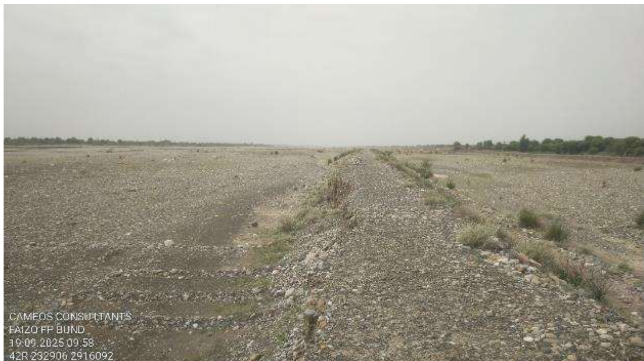
Figure-3-2: Alluvial/riverbed deposits along the washed-out bund.
